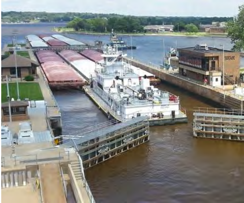
Figure 3 Example of a Lock
