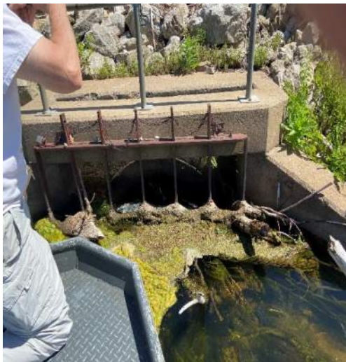
Figure 5 Single 3-foot culverts as observed on August 4, 2022
