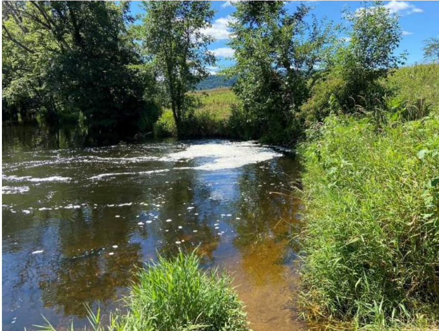
Figure 4 Three 4-foot culverts as observed on August 4, 2022
