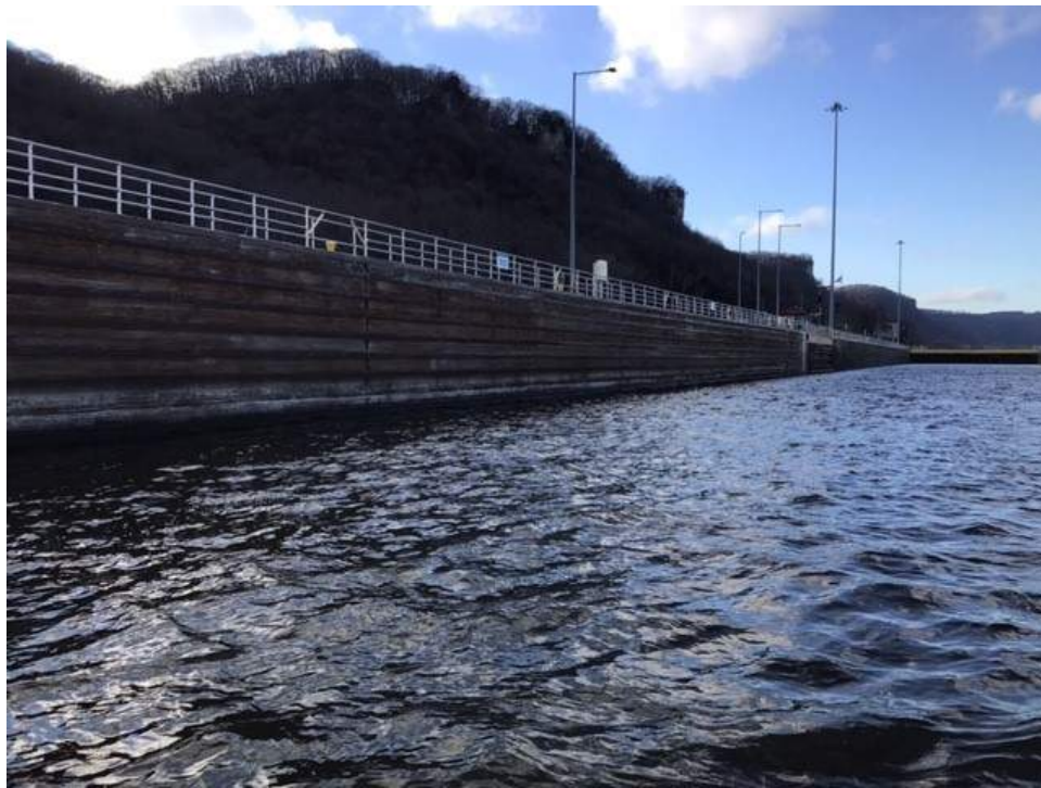
Figure 5 - Land Wall: Overall Good Condition
