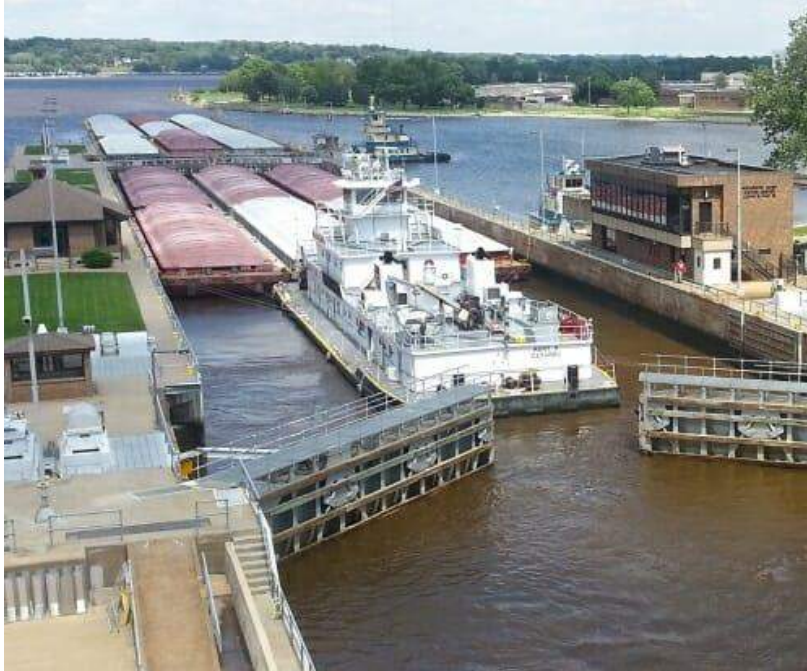
Figure 3 Example of a Lock
