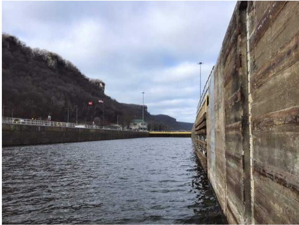
Figure 4 - I-Wall: Overall Good Condition
