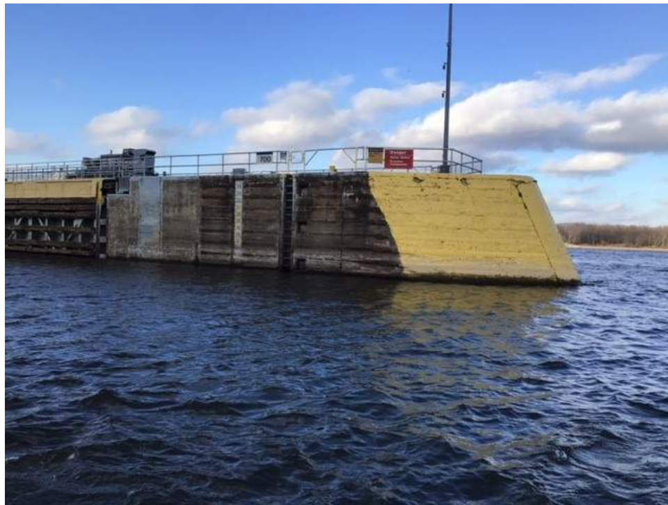
Figure 3 - I-Wall: Overall Good Condition
